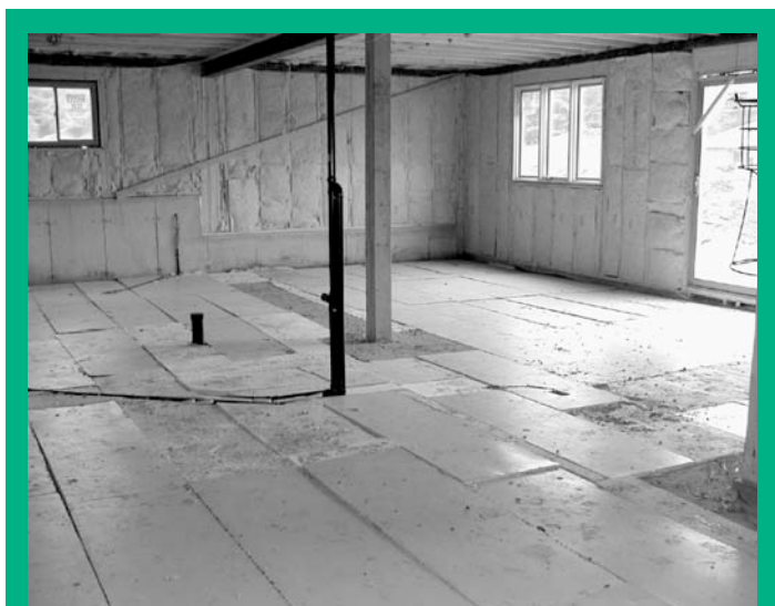
This underslab insulation made from scrap insulated steel door window cutouts scored highest in the CMHC test.
